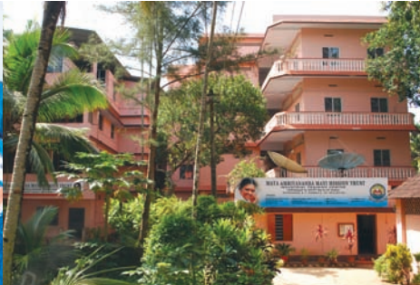
Industrial Training Centre, Karunagappally
